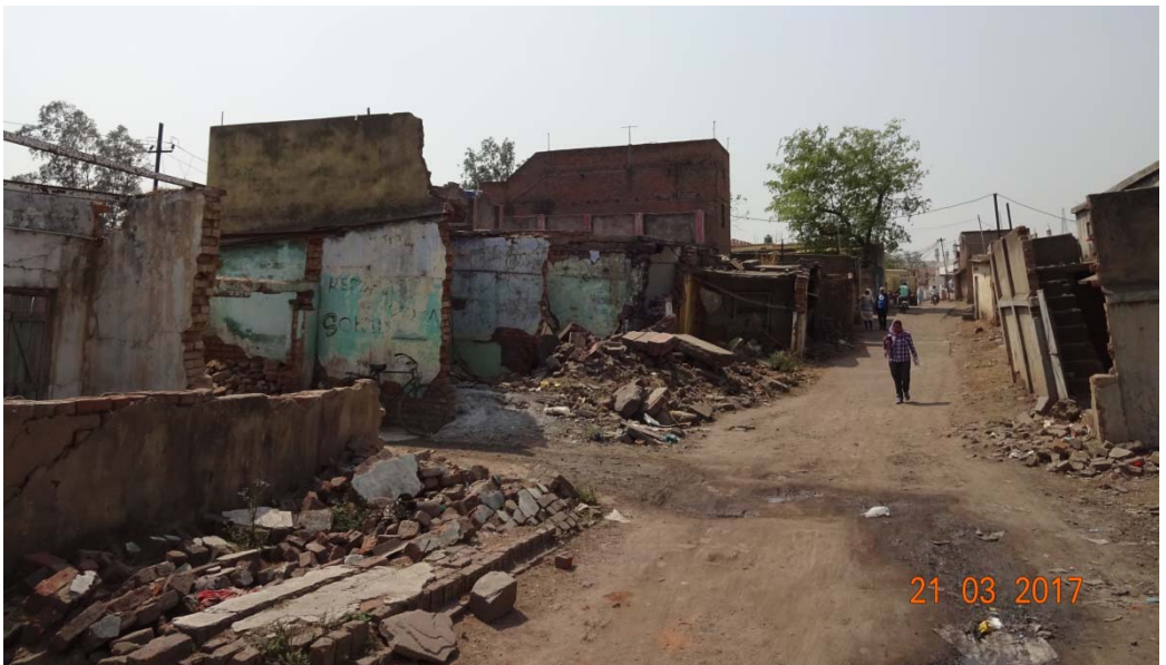
Jogta colliery (Jharia) – Houses abandoned due to coal fire risk – no safer place offered!
